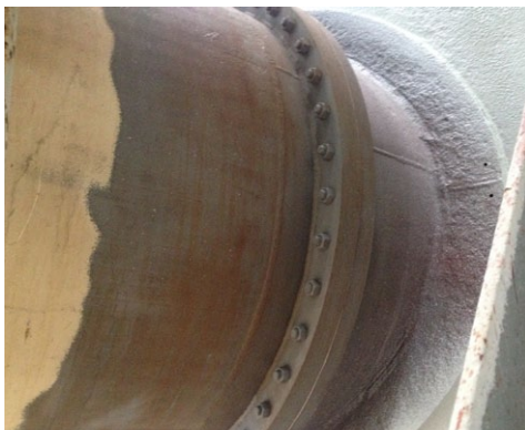
52" flange prepared for application
