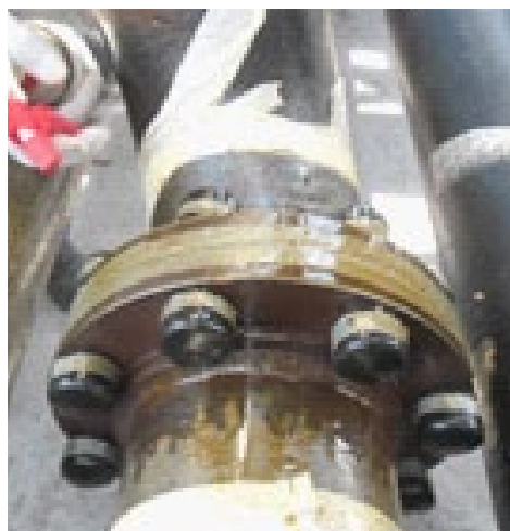
Application of Belzona 8411
