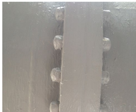
First coat of Belzona 3411
