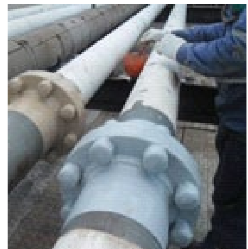
Application of Belzona 3411
